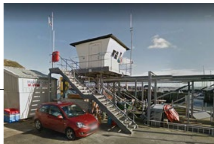
Building 6 (Watch keepers office) Building to remain
