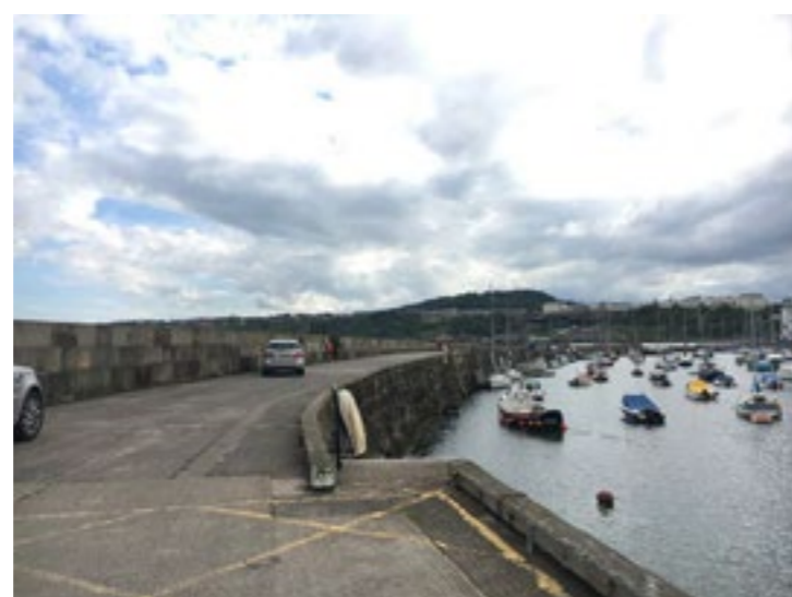
Lack of public realm and lighting on North Pier.
